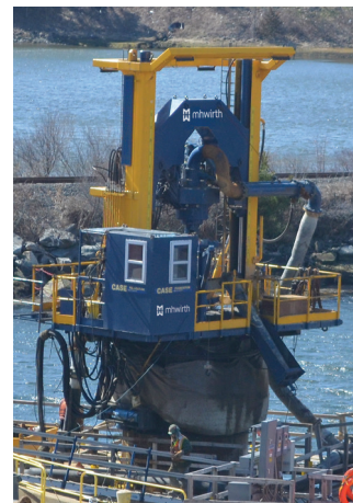
USA/New Hampshire/Maine – Sarah Mildred Long Bridge PBA 933/3 000/300 for the foundation of 29 piles to replace the existing bridge; with a drilling diameter of 2.9 m and depths of up to 50 m
