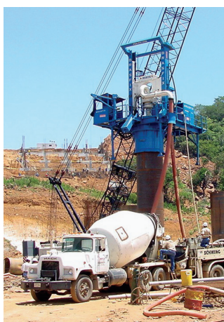
Venezuela – Orinoco Bridge Three PBA 818 and one PBA 612 to install 156 piles (bridge length: 3.2 km), with diameters of 2.4 m and 1.8 m, and depths of up to 60 m
