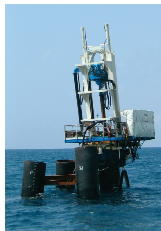
Australia – Tanker terminal PBA 612/2 000/200 for raker piles at an inclination of up to 1:3, with drilling diameters of up to 1.25 m and depths of up to 50 m
