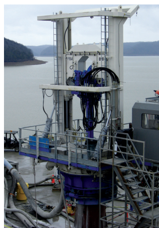
USA/Kentucky – Wolf Creek Dam PBA 818/2500/300 for a cut-off wall, with a drilling diameter of 1.27 m, depths of up to 90 m, rock strengths of up to 150 MPa
